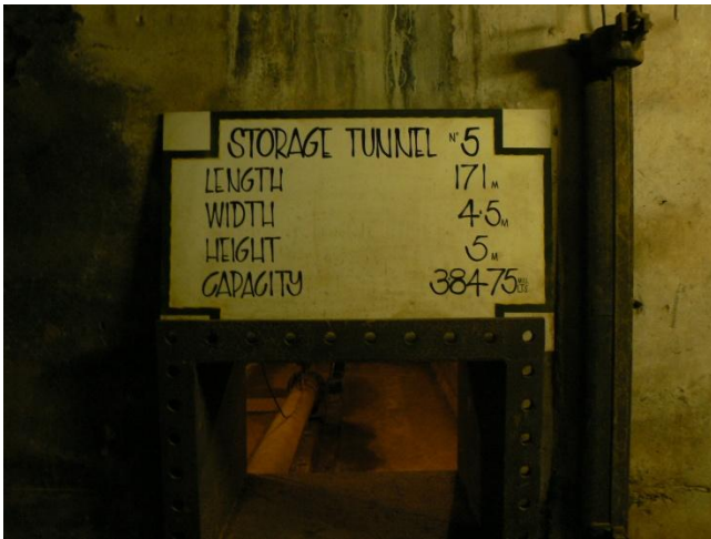
The measurements above are in metres with the capacity 3.8575 million litres.
